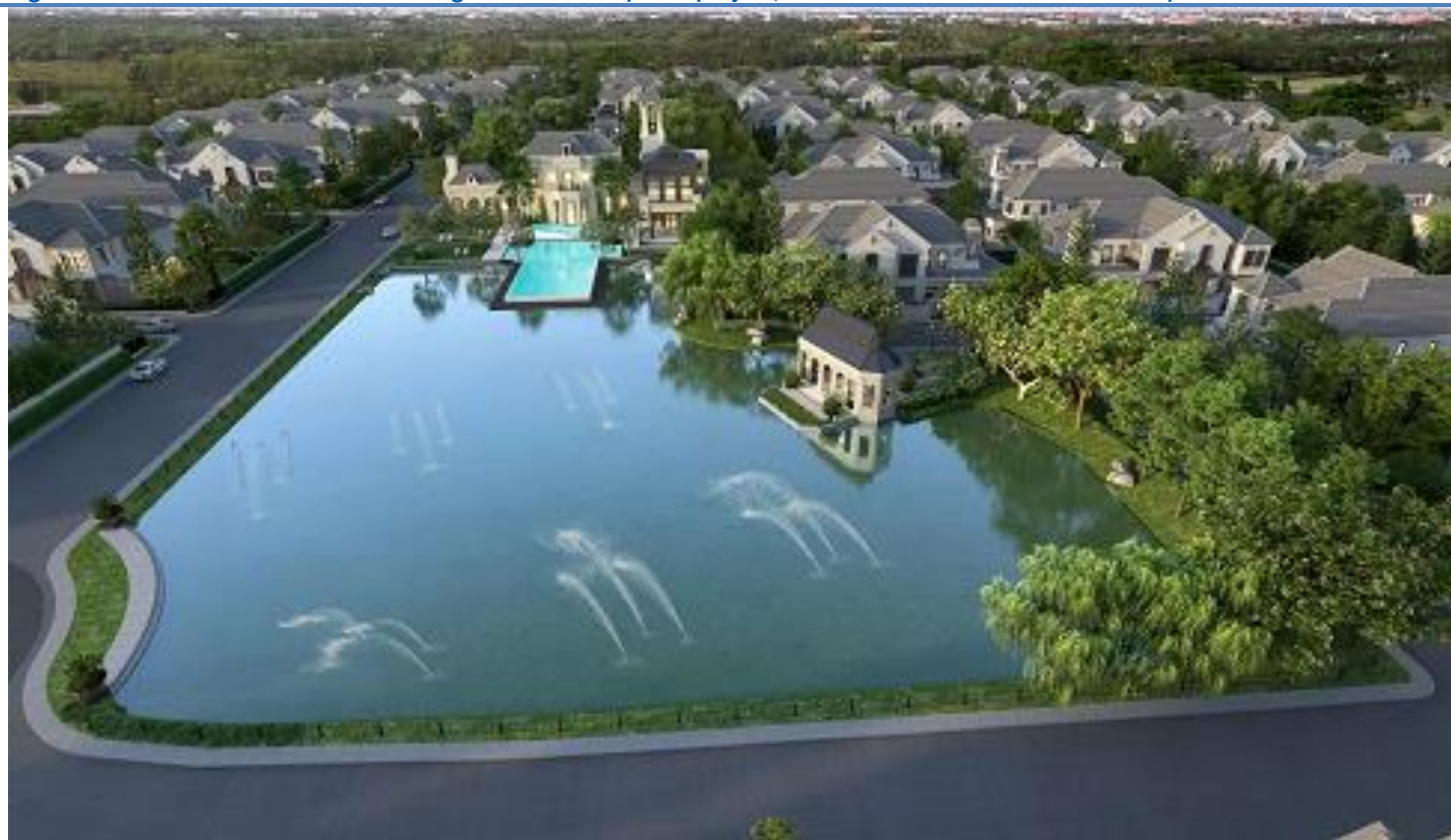
Figure 2: An aerial view of Nantawan Bangna km 15 luxury SDH project, which was launched in mid-February
